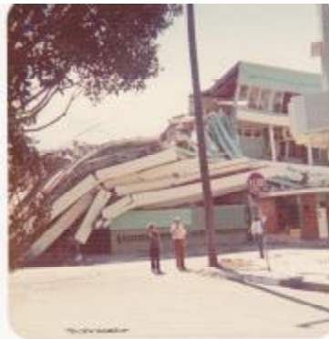
Collapsed multi story apartment building where many people were killed and bodies not yet recovered.
